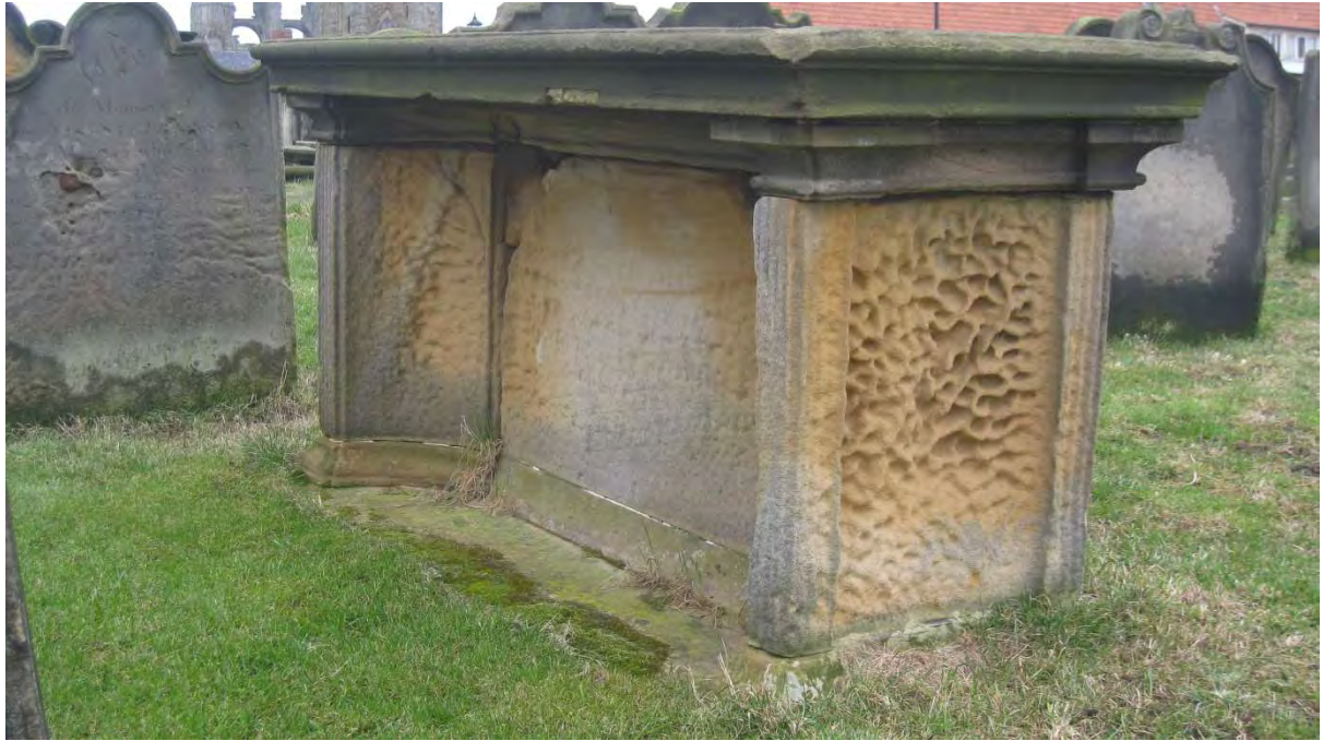
Photo 3 Typical weathering of the Middle Jurassic sandstones overlying the Whitby Mudstone Formation. The old graveyard at St. Mary's church, Whitby.
