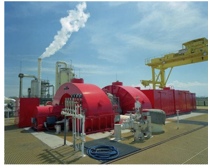
Warmtekrachtpompen (bron: sites.google.com/site/renewablefeed/geothermal)
